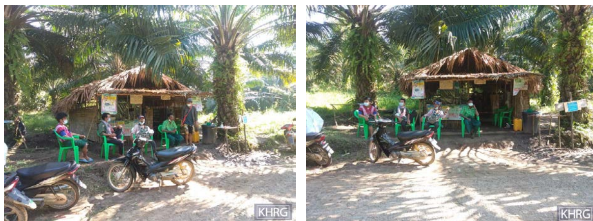
These photos were taken on 7 th November 2020 in the S'Tain area, Lenya Bokpyin Special Area, Mergui-Tavoy District. They show the COVID-19 screening checkpoint built by the local villagers with support from the KDHW. [Photos: KHRG]
