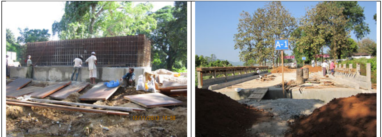
The photo on the left was taken on December 11 th 2013 in the northern part of Ma Htaw village in Ma Htaw village tract, Dwe Lo Township, Hpapun District. It shows workers constructing steel frames to be used as the foundation of Nyi Naung Bridge. The photo on the right was taken on December 27 th 2013 in Ta Kun Taing village in Meh village tract, Bu Tho Township, Hpapun District. The photo is of the completed T'Kun Taing Bridge. [Photos: KHRG]
